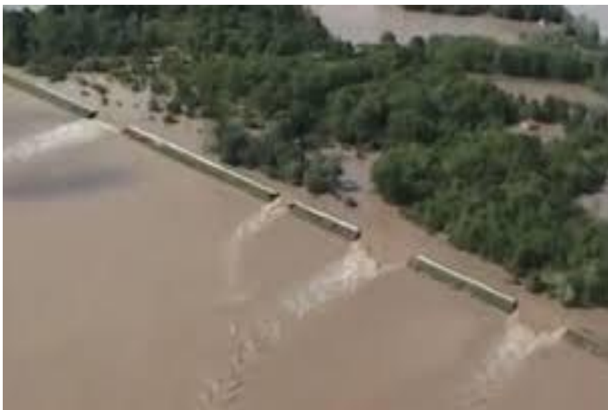
Picture 1. Damaged parts of the Sava river embankment 2014
