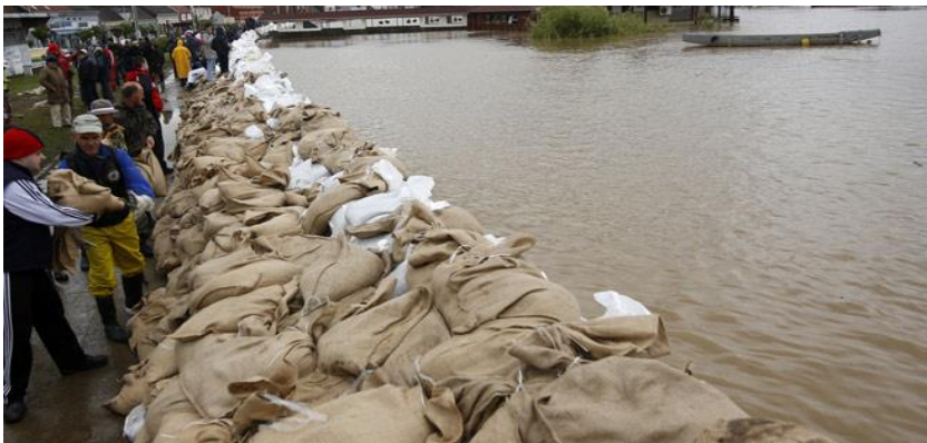
Picture 3. Construction of the Sava river embankment 2014
