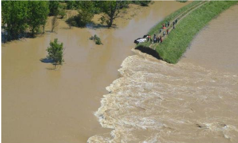
Picture 2. Damaged parts of the Sava river embankment 2014
